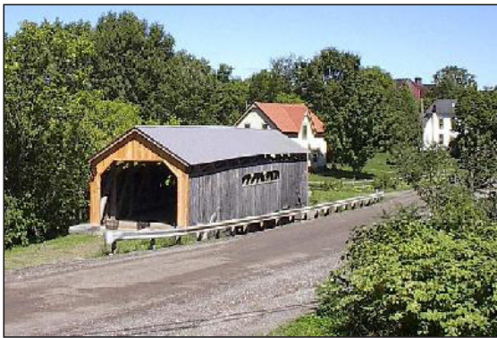
Now restored, Westford's Browns River Bridge in place.
