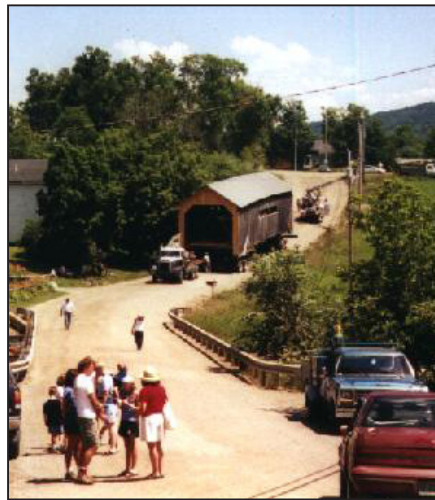
Westford bridge moving down the road to its new location.
